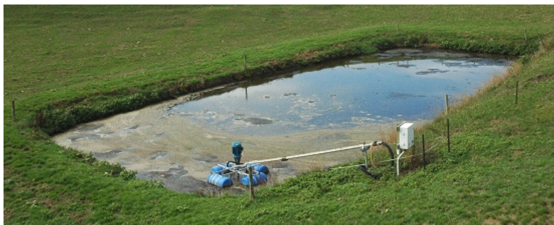
Figure 2. Effluent pond and pump
